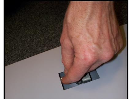
Using your other hand take hold of the locking bar and try to guide the bar onto your screwdriver (this can be tricky until practised)
